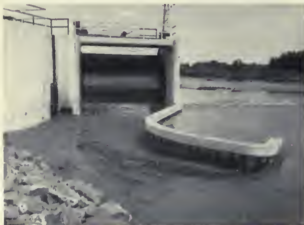
RECEDING FLOOD on Republican River (below) shows curved steel sheet piling wall at Superior headworks. Right, silt bed in model of Courtland Canal. Below, E. J. Carlson (center) adjusting sluice gate on model of Courtland headworks, O. S. Hanson (right) regulating sand feed into dam as R. S. Brown (left) checks sediment samples. Two photos at right by G. F. Breitung, Branch of Design & Construction, Denver, Colo. Photo below by R. Boyce, Bureau of Reclamation.
